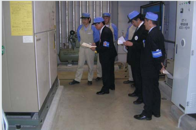
Members making an “energy-saving diagnosis”
