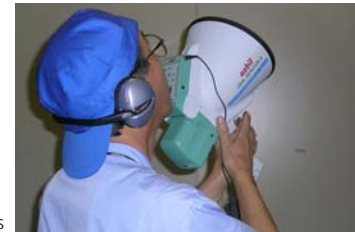
Inspection of air leakages
