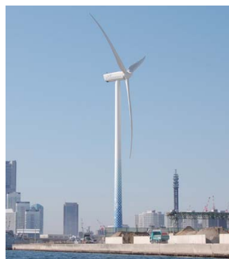
Hama-Wing (Yokohama City wind power plant)
