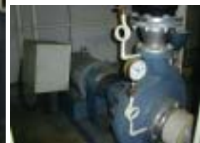
Pump inverter equipment introduced at the Mito Plant
